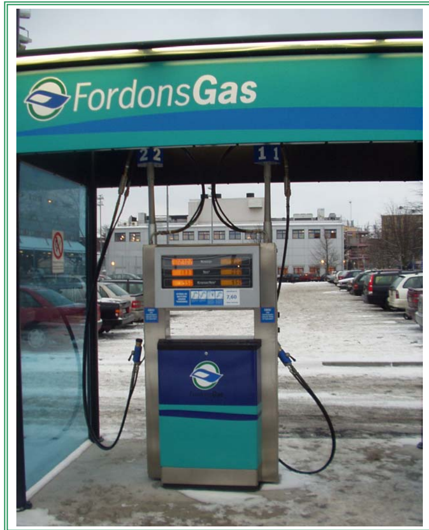
(Biogas fuelling station for bi fuel cars, Göteborg, Sweden)
